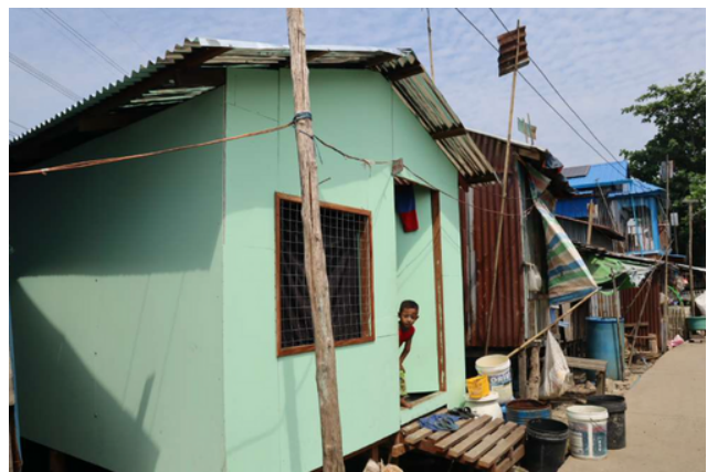
Shwe Htu's house after
